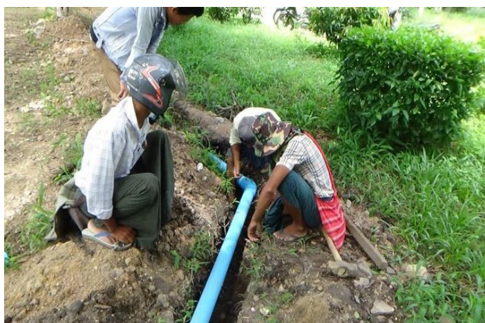
Figure 11 Connecting water pipes (by FRI)
